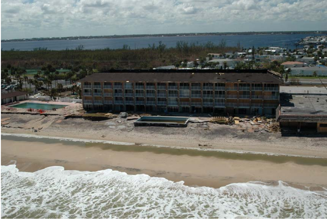
Photo 30: Erosion and Damage, South Hutchinson Island (R106)
