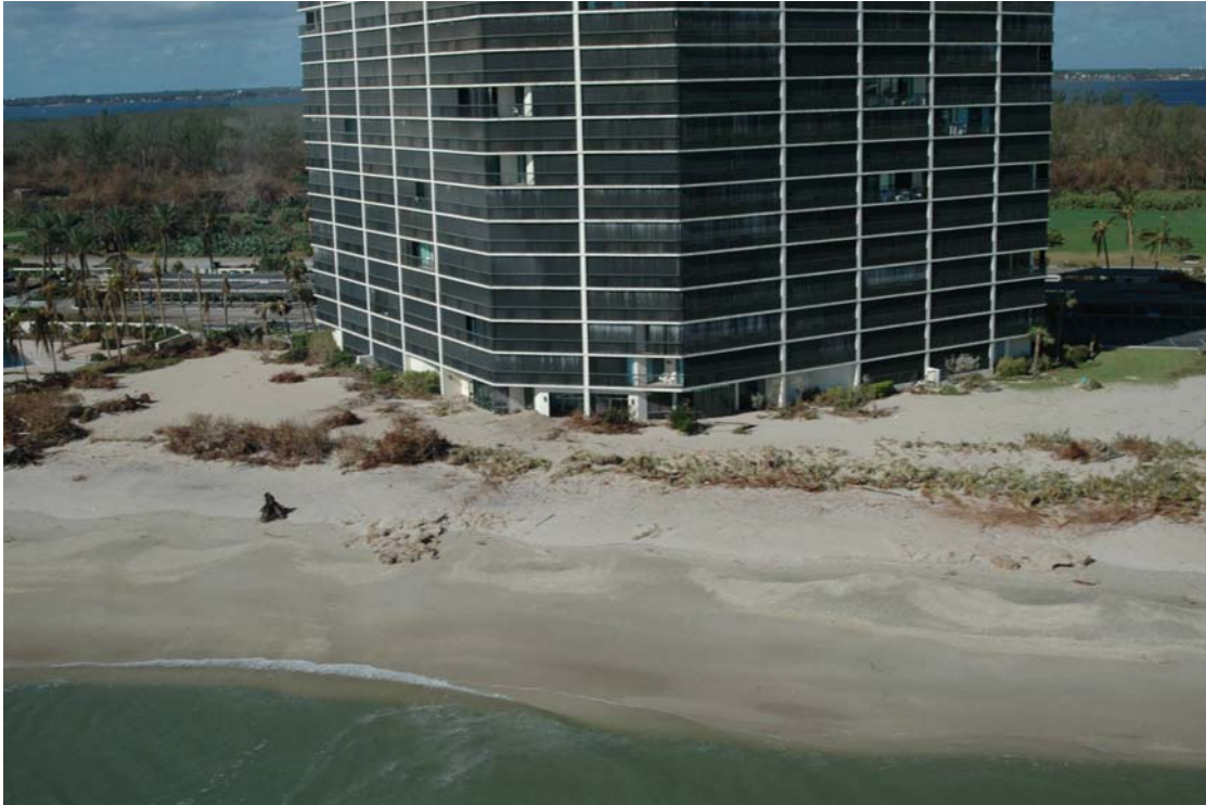
Photo 26: Dune Erosion and Washover, South Hutchinson Island
